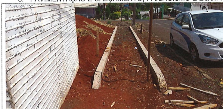
Guia de concreto moldada in loco
