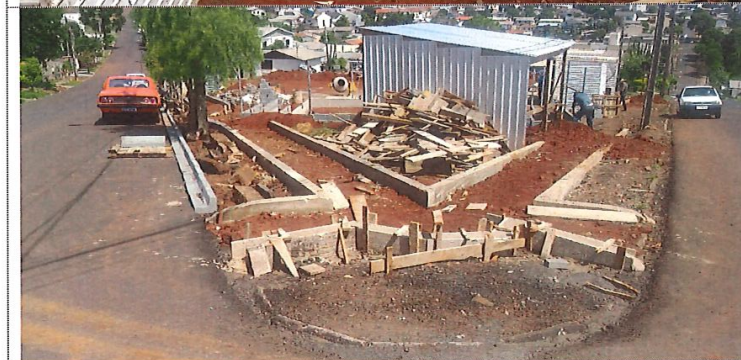
Guia de concreto moldada in loco
