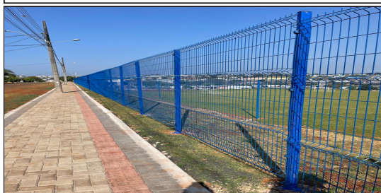
7 | alambrado e escadaria
