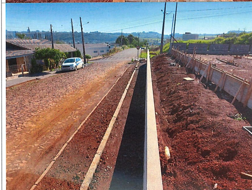
Guia de concreto moldada in loco
