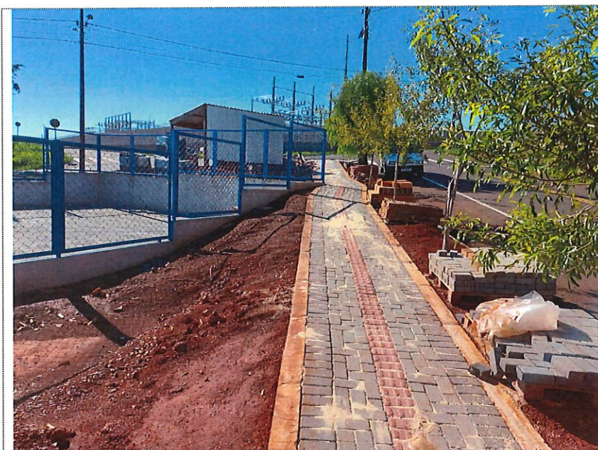
Guia de concreto moldada in loco
