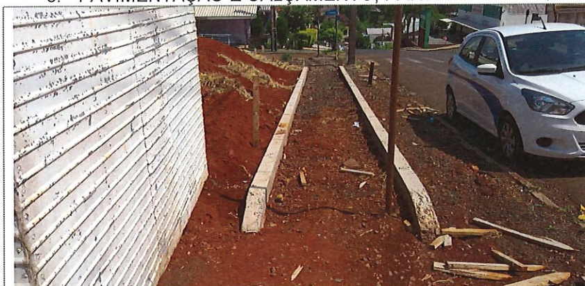
Guia de concreto moldada in loco
