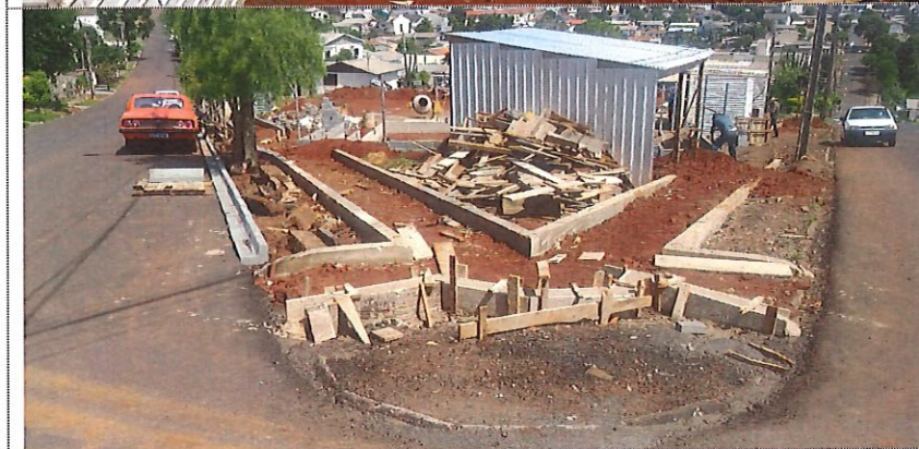
Guia de concreto moldada in loco
