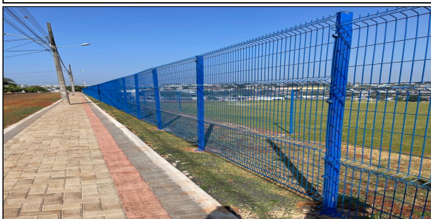
7 | alambrado e escadaria
